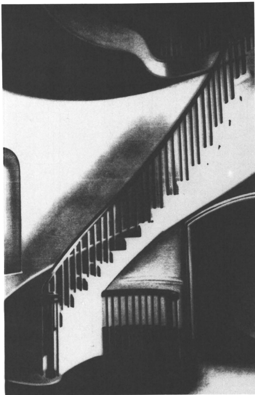
Figure 2. Views of "Stairway 1910, Richmond", by Lowell Nesbitt
